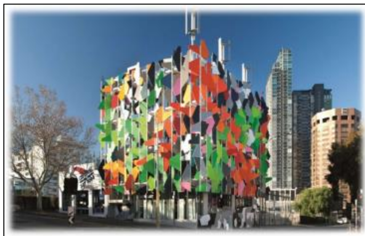
Figure 4: Pixel building foldable façade plates for optimal shading and ventilation
