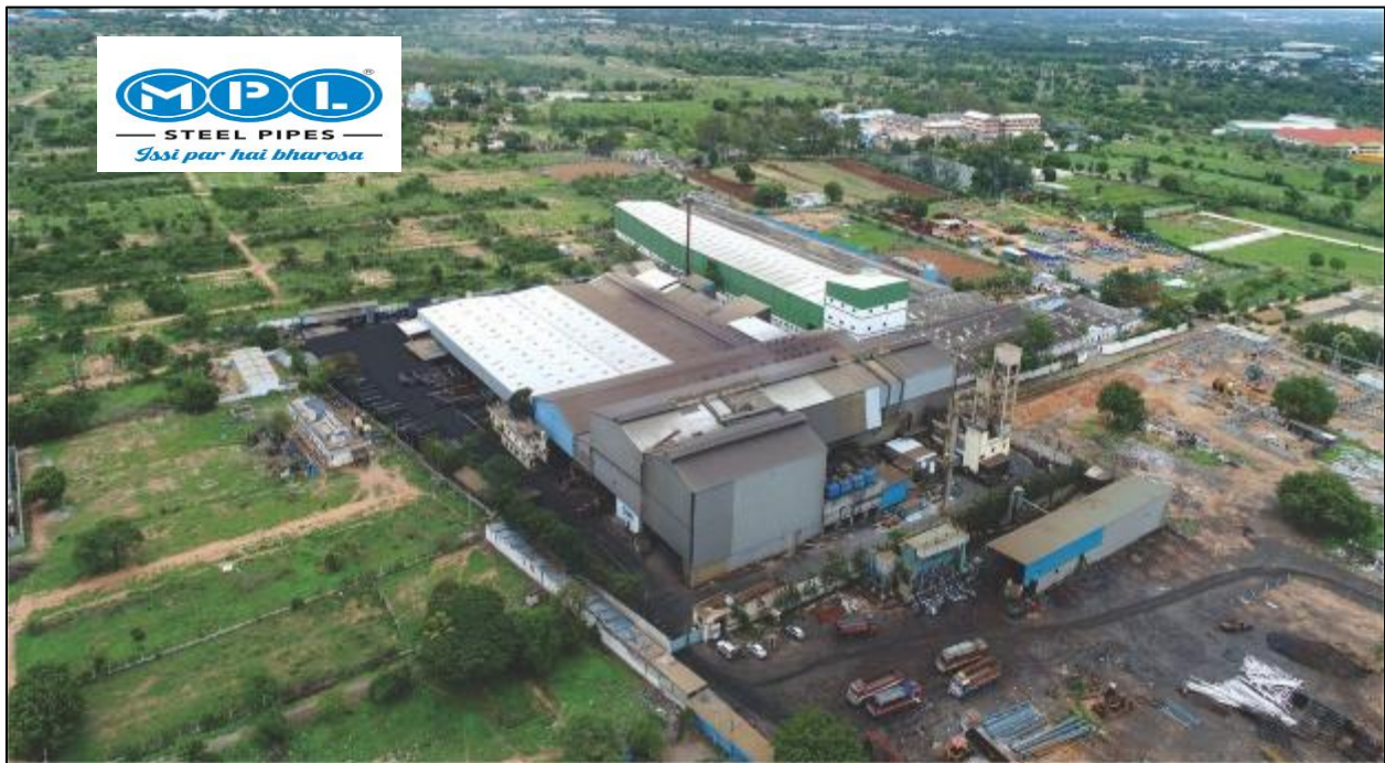
Figure 1 MPL Steel Plant
