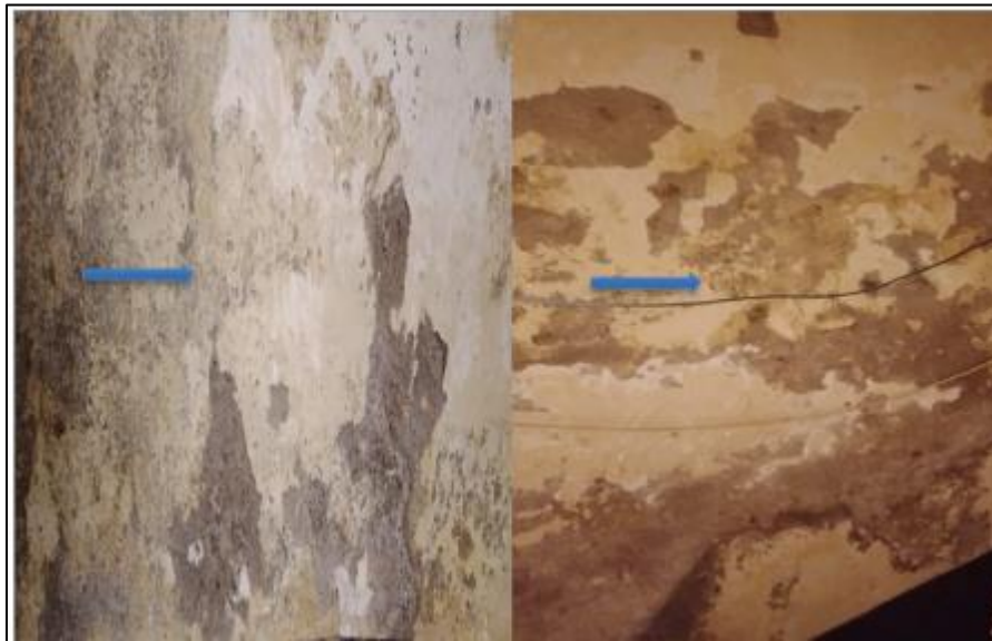
Figure 3 Significant domestic mold infestation and severe wall dampness identified as the primary antigenic source
