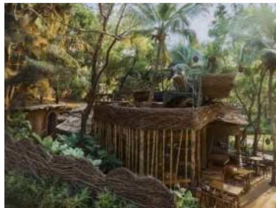
Figure 5 Como Agua showcases the use of Lantana Camara, as a primary building material.
