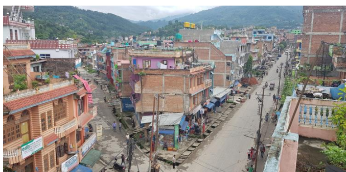
Figure 5 New building with R.C.C structure
