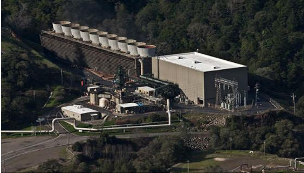
Figure 11 Power plant within the Geysers (Calpine)
