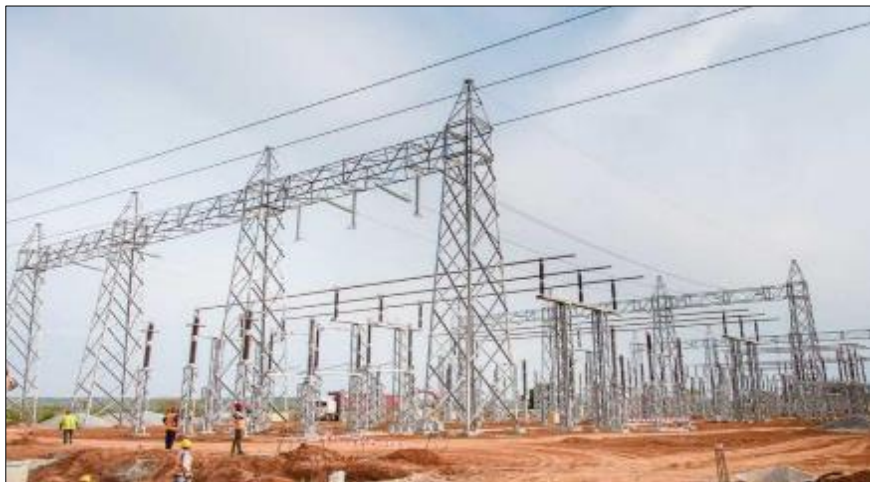
Figure 3 Electrical Grid Infrastructure (Google Photos)
