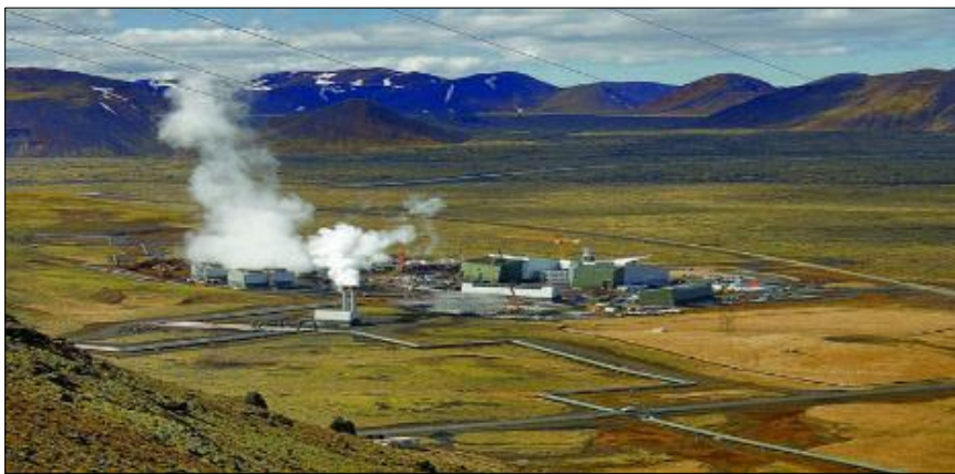
Figure 4 Hellisheiði Geothermal Power Project, Hengill (Renewable Technology)
