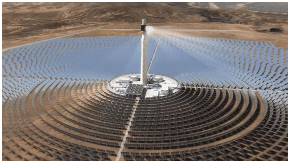
Figure 10 Noor Ouarzazate solar complex (Safaa Kasraoui)
