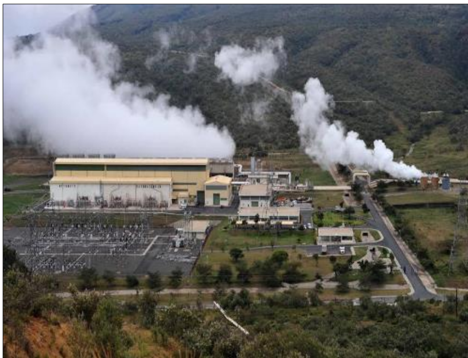
Figure 8 Olkaria Geothermal power project (credit: KenGen)
