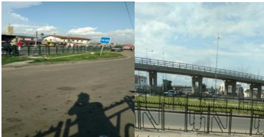
Figure 6 The Newly Constructed Road and Fly Over in Sodiko
