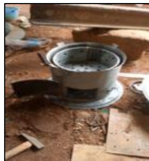
Figure 7 Assembling the various parts of the primary- and secondary-source cookstove
