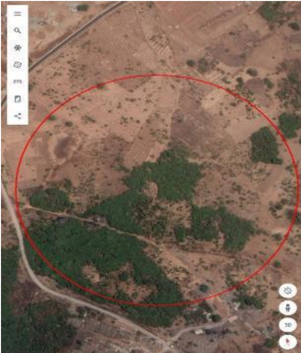
Figure 5 Buffered of River Park dumpsite
