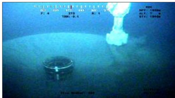
Figure 9 Phase 2: 26" drill outlet
