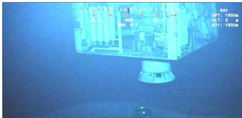
**Figure 15** Phase 2: Approach of the BOP to the wellhead
