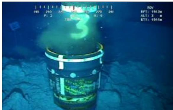
**Figure 11** Phase 2: 20" shoe passing the ABP
