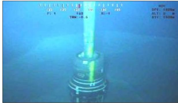
**Figure 13** Phase 2: Attach the 20-inch high-pressure housing (AAP) to the low-pressure housing (ABP)
