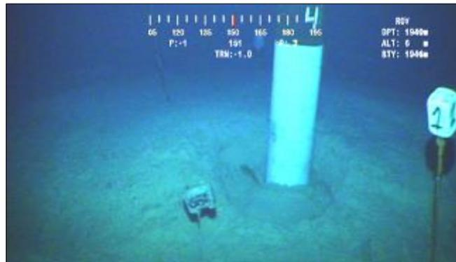
**Figure 3** Phase 1: Marking the column in relation to the mud line
