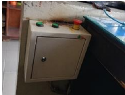
Figure 3 Fire Alarms at PT Wijaya Karya Beton Tbk. Pasuruan
