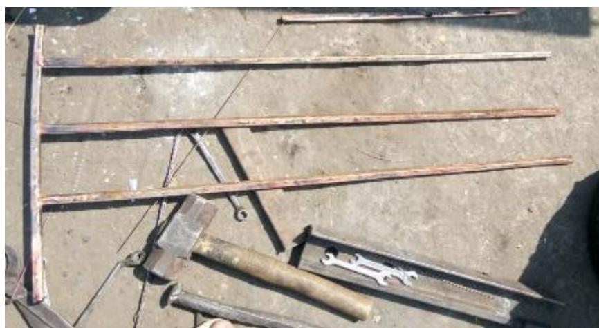
Figure 4 Assembly of Solar Water Heater Pipe
