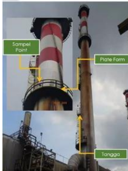
Figure 1 Existing condition and sample point location of the stack
