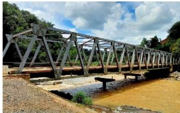
Figure 1b Manupali steel truss bridge
