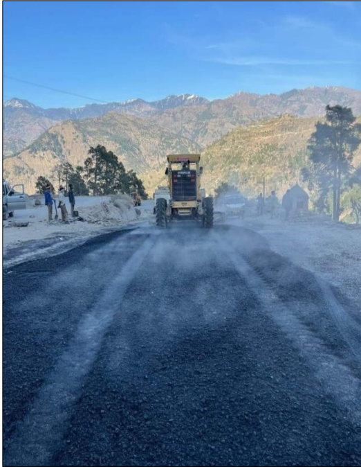
Figure 5 NH-44 at Kashmir section
