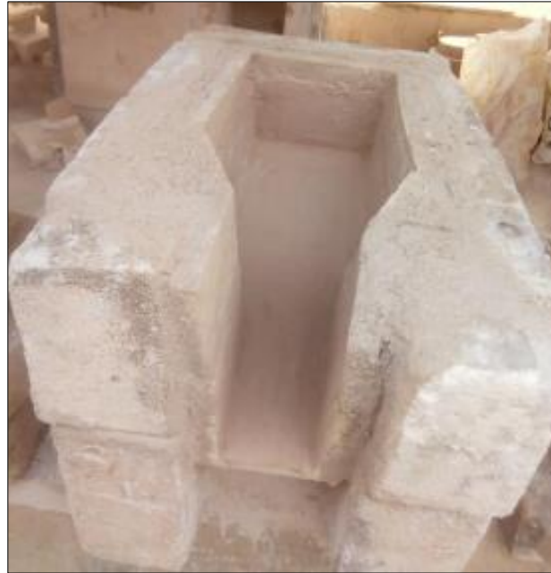
Figure 7 The Furnace Base Wall Lined with the Monolith
