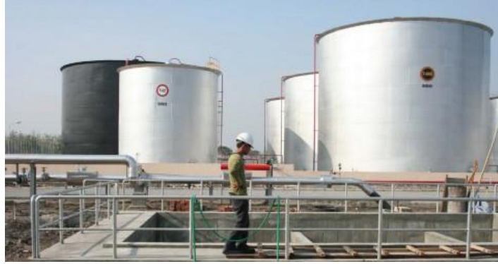
Figure 2 Cepu Main Fuel Tank 401
