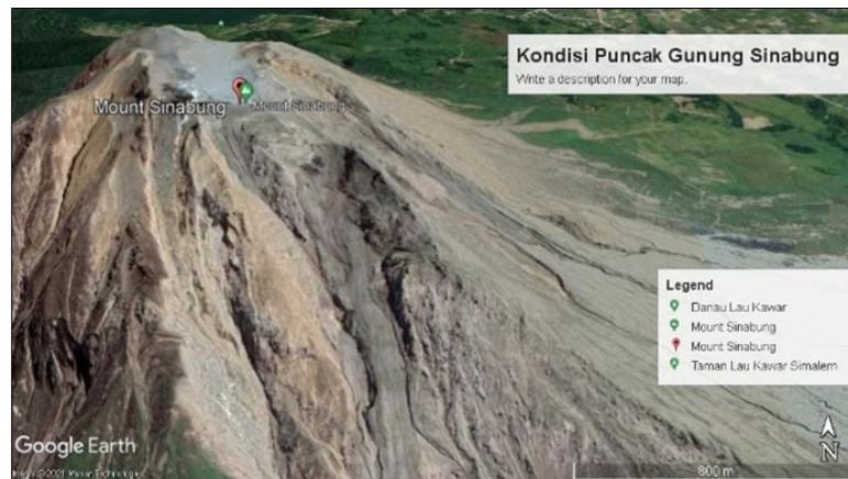
Figure 11 The condition of Peak Sinabung which landslides after eruption
