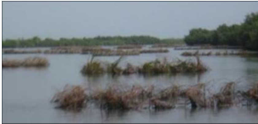
Figure 13a Acadjas parks still called Amédjrotin installed in the Ahô channel
