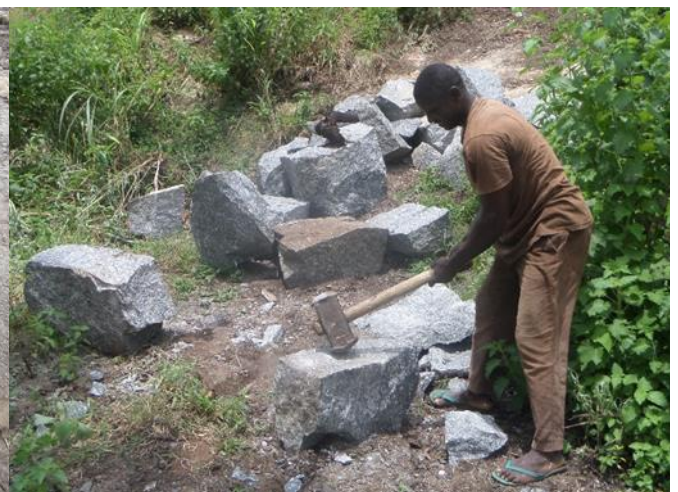
Photo1 b Stripping operation
